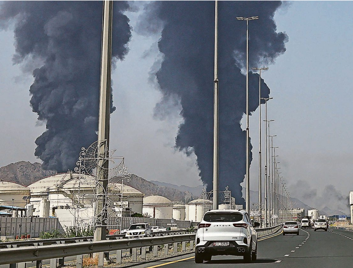
Smoke rises from the direction of an energy installation in the the United Arab Emirates’ Fujairah emirate on March 14. Some oil-loading operations were suspended, sources said. AFP VIA GETTY IMAGES
