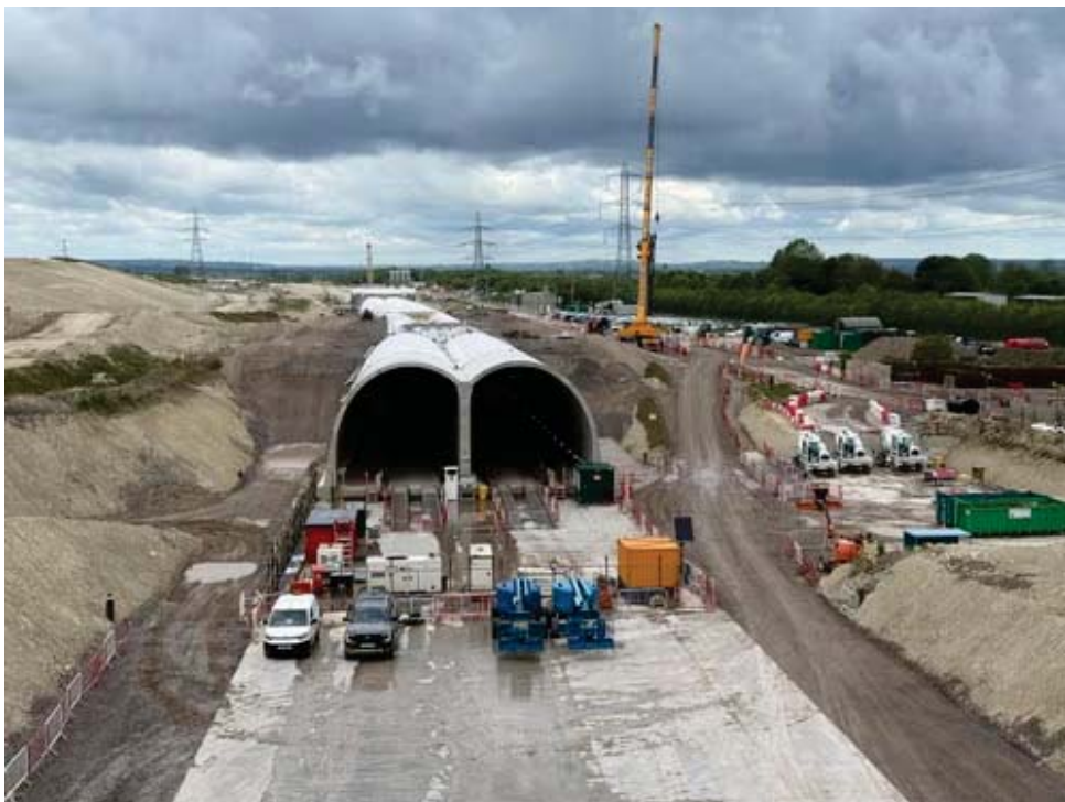
Work continues on the mile-long Wendover tunnel (Supplied)
