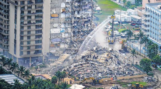
The remains of the Champlain Towers South in Surfside, Fla., in June 2021. The collapse caused the deaths of 98 people.
