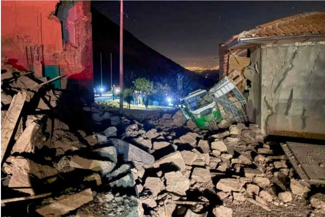
Dozens of homes were destroyed and 18 damaged in Peru, affecting around 300 residents (AP Photo/Jhefry Sedano)
